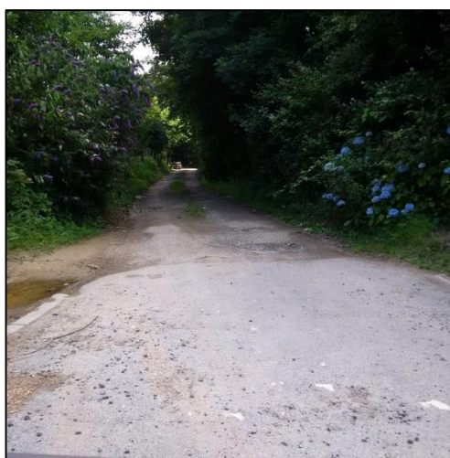
Figure 3.23: Possible access location for chainage 7200m – 8100m.
